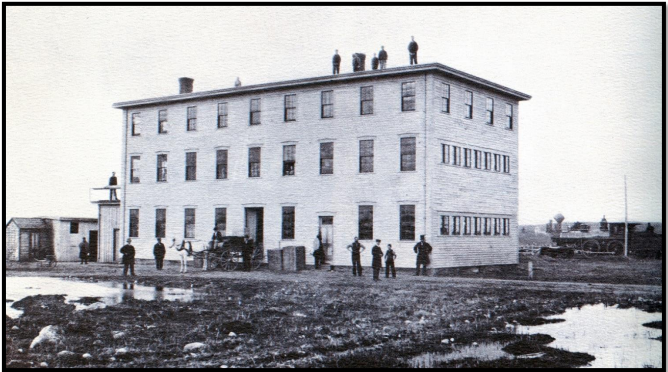
Building Carter's first mill, on the corner of Highland Avenue and West Street, 1865
